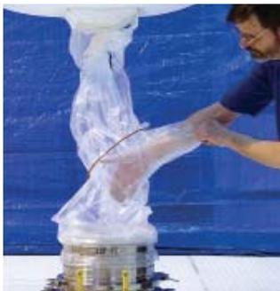
Attach liner then bag out stub
