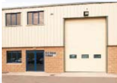
ILC Ireland facility
